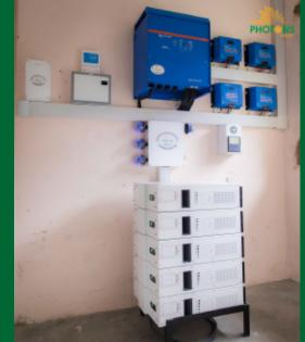
Project Discription CRADLE OF LOVE (USA RIVER) 16.8kWp Solar PV system 24.75kWh battery bank (Lithium Battery)
