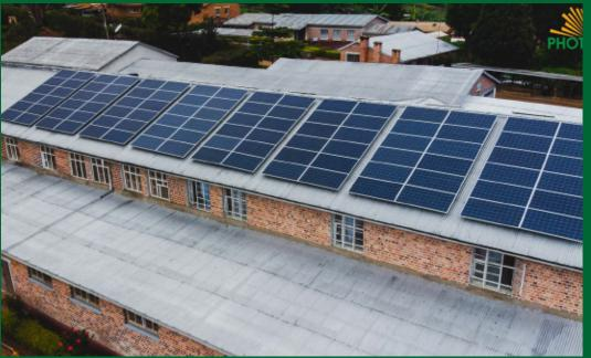
Project Discription LITEMBO HOSPITAL- GRID TIE SOLAR PV SYSTEM 32 kWp Solar PV system Offest most of the day time energy consumption Batteryless solar PV system
