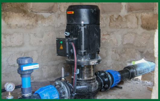
Project Discription SAME- SOLAR WATER PUMP SYSTEM 10m Total head 600m Horizontal Distance 900000 liters per day 16kWp Solar PV System pump type lorentz.
