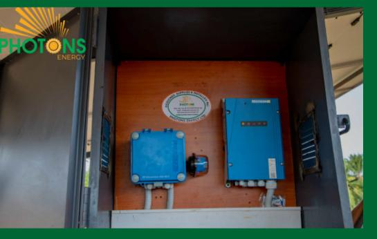
Project Discription SUNUKA KIGOMA – SOLAR WATER PUMP SYSTEM 20m Total head 400m Horizontal Distance 230000 liters per day 8.1kWp Solar PV System pump type lorentz.
