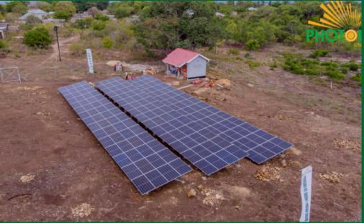
Project Discription Kokota Islet in Pemba - Zanzibar 80.1kWp Solar PV system 150kWh battery bank Provides 100% of the whole Islet Electrical Energy
