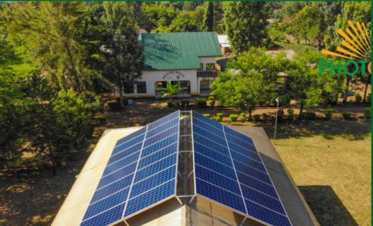
Project Discription MAWELA VTC – GRID TIE SOLAR PV SYSTEM 10 kWp Solar PV system Offest most of the day time energy consumption Batteryless solar PV system
