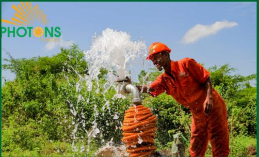
Project Discription GITOYA BARIADI – SOLAR WATER PUMP SYSTEM 190m Total head 6Km Horizontal Distance 150000 liters per day 28kWp Solar PV System pump type lorentz.
