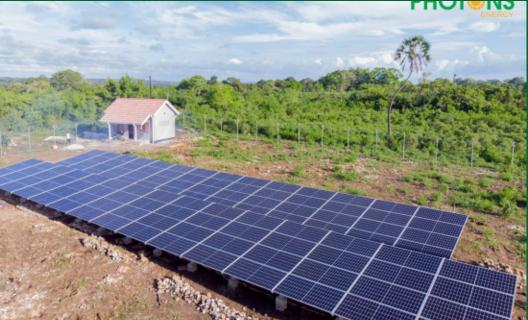
Project Discription Njau Islet in Pemba - Zanzibar 51kWp Solar PV system 99kWh battery bank Provides 100% of the whole Islet Electrical Energy
