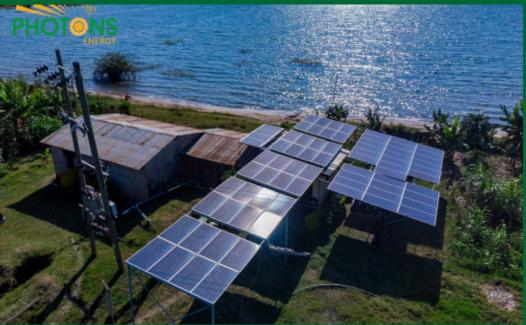
Project Discription SHIRATI HOSPITAL- SOLAR WATER PUMP SYSTEM 80m Total head 3Km Horizontal Distance 150000 liters per day 18.8kWp Solar PV System pump type lorentz.
