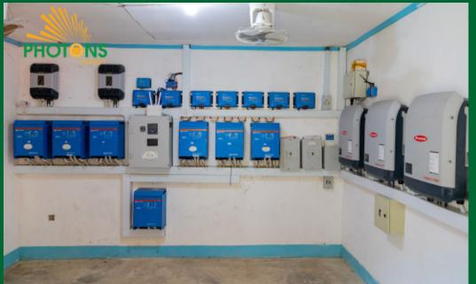
Project Discription Shirati KMT Hospital 84kWp Solar PV system 480kWh battery bank Provides 100% of the Hospital Electrical Energy
